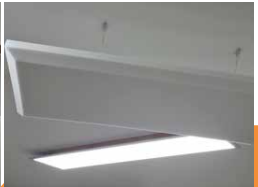
INSTALLED Now repeat for the remaining ceiling panel
