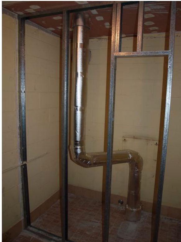
Figure 3.4 Pipe Lagged with Acoustic Pipewrap
