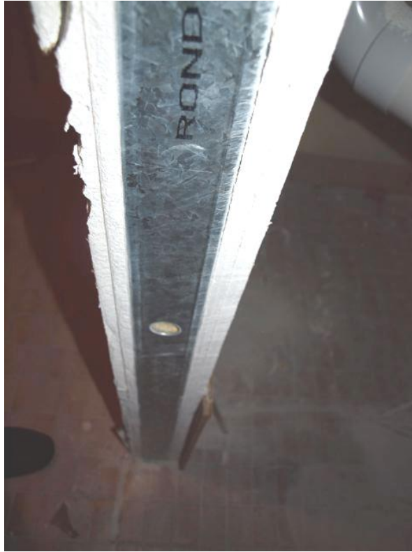
Figure 3.4 Pipe Lagged with Acoustic Pipewrap
