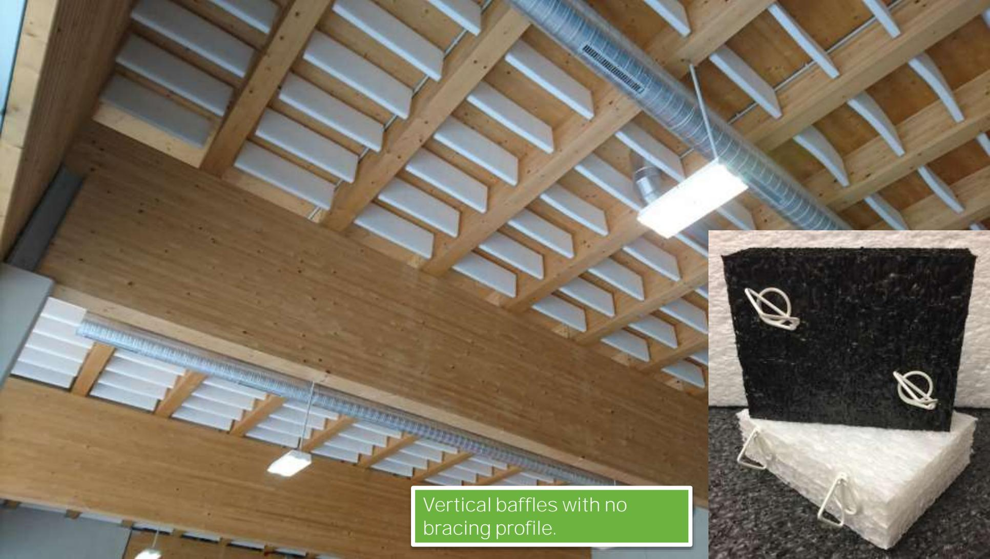
Vertical baffles with no bracing profile.
